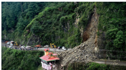
Figure 4: Landslides caused by excessive rainfall caused damage and disrupted traffic.
